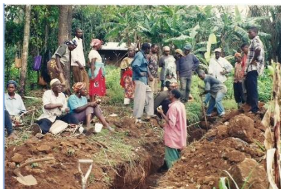
Photo 1: Women Participation in Digging Water Pipeline in Bambili
