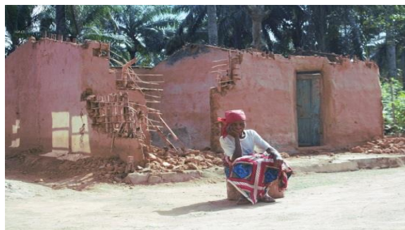
Plate 5: Before FEYRep Intervention
