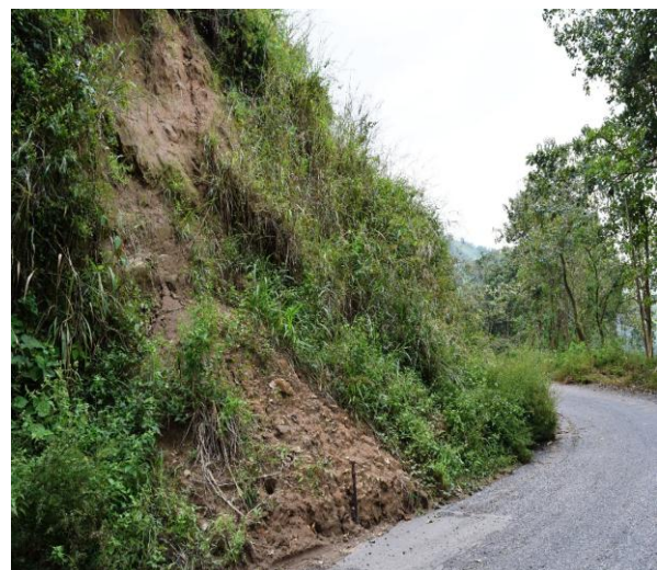
Figure 6d: Landslides of Befang Forest
