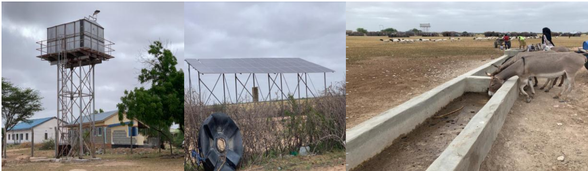
Plate 3 Newly constructed Water Troughs, Storage Facility and Solar Panel in Goreale Ward through CCCF (Field Work, 2020)
