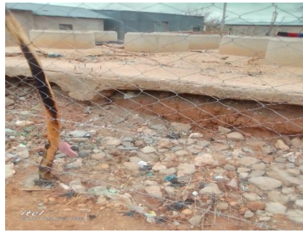
Plate 4: Raised House Under Construction As Flood Adaptation Strategy in Madogo Ward, Kenya.
