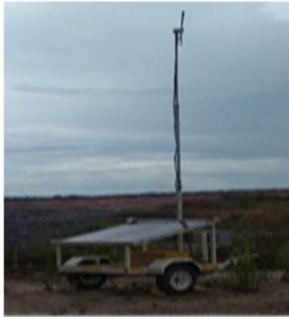
Figure 5: FAP08 HIA Access point
