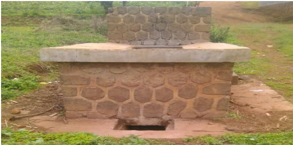
Figure 2: A stand tap constructed in Presbyterian Quarter
