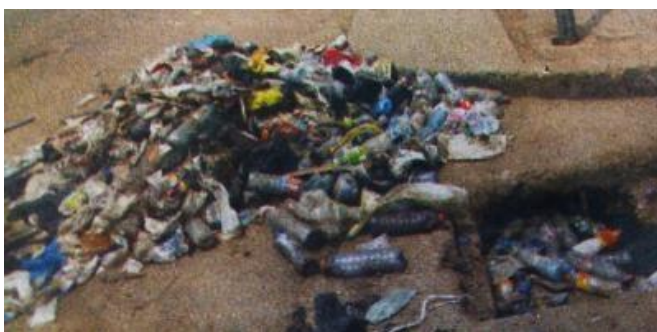
Plate 4: Packaging waste choking the gutter
