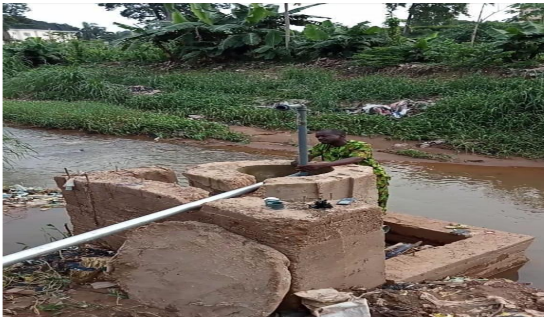
Plate 1. Sump/ Infiltration Structure
