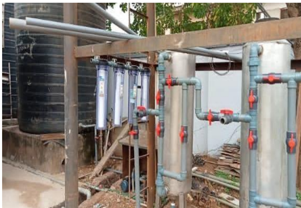
Plate 2. Local Water Treatment Plant
